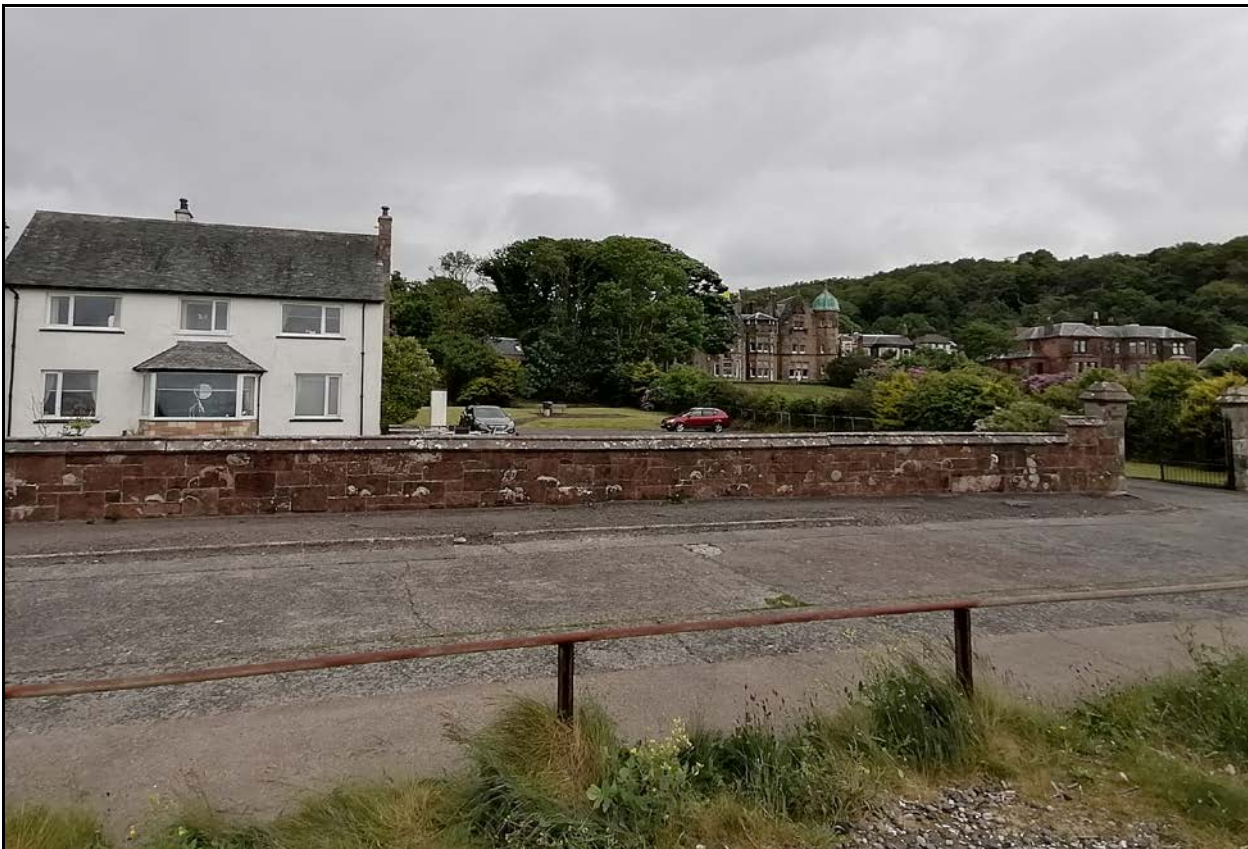
The site as viewed from Wemyss Bay Road
